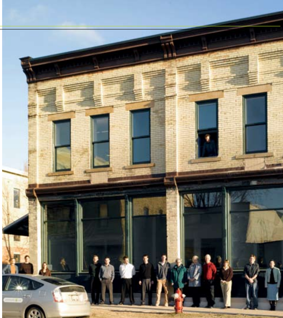
Midwest Environmental Advocates' office was converted using green building principles.
