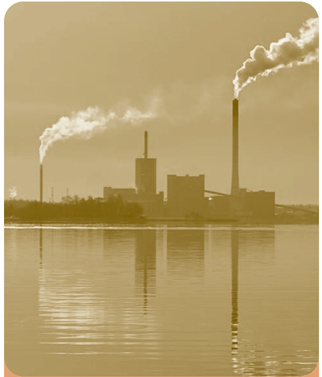
Midwest Environmental Advocates is working to reduce air pollution from smokestacks like these.
